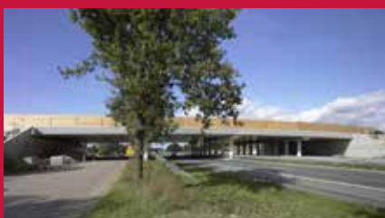
Wildlife Crossing Weerterbergen
